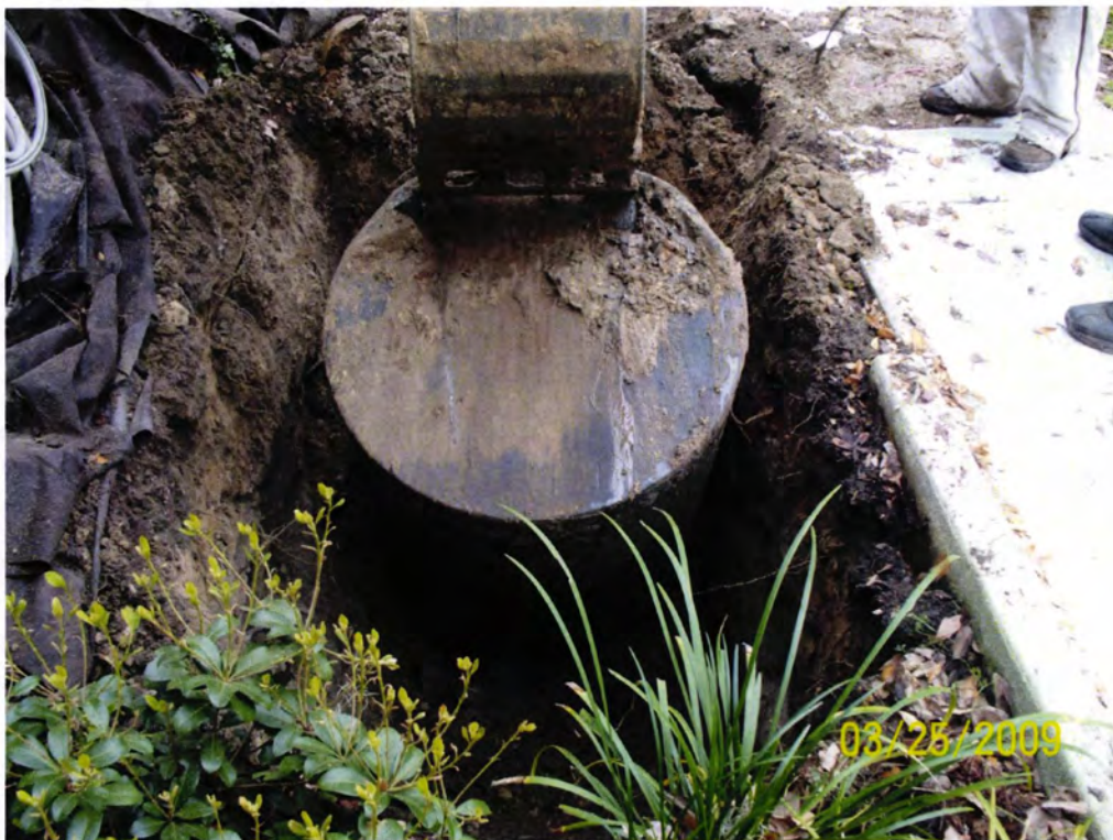
Picture 2: UST 160Cypress during removal from the excavation.
